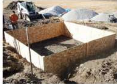
Frame for RVF wetland cell liner.
