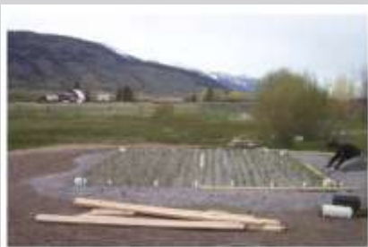
Planting completed May 26, 2010
